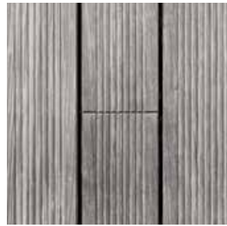
Gradual greying of MOSO® Bamboo X-treme® over time: new, non-weathered decking (left), after 3 months of weathering (middle) and after 18 months of weathering (right).
